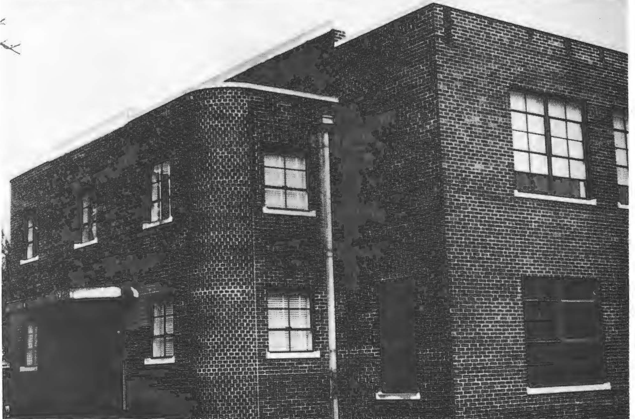
Library and Industrial Arts Building
